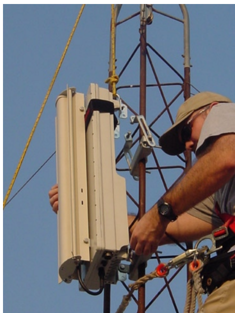
Solectek WiMAX base station installation in Indiana.
